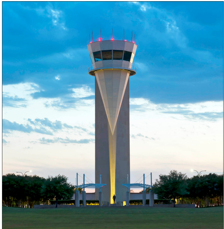
Alliance Fort Worth (AFW) Airport.
