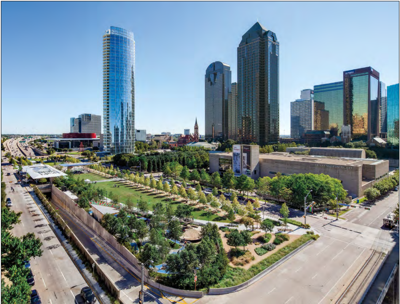
The Klyde Warren Park in Dallas opened in 2012. It was built above the Woodall Rodgers Freeway. Photo courtesy of Thomas McConnell
