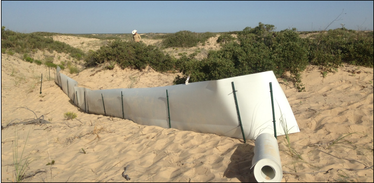
Figure 1. Construction of temporary enclosures 1 and 2 with Animex® fencing material.
